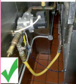
Restraining wire attached to the wall
