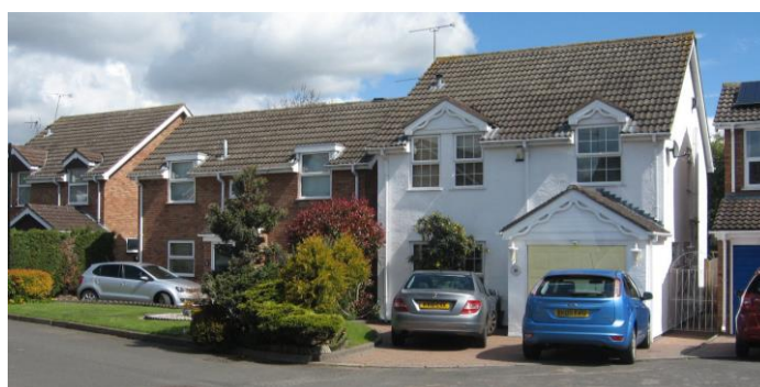
View of typical housing in Roman Way
