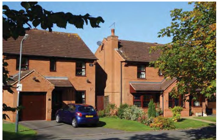
Shared driveway off Glasshouse Lane
